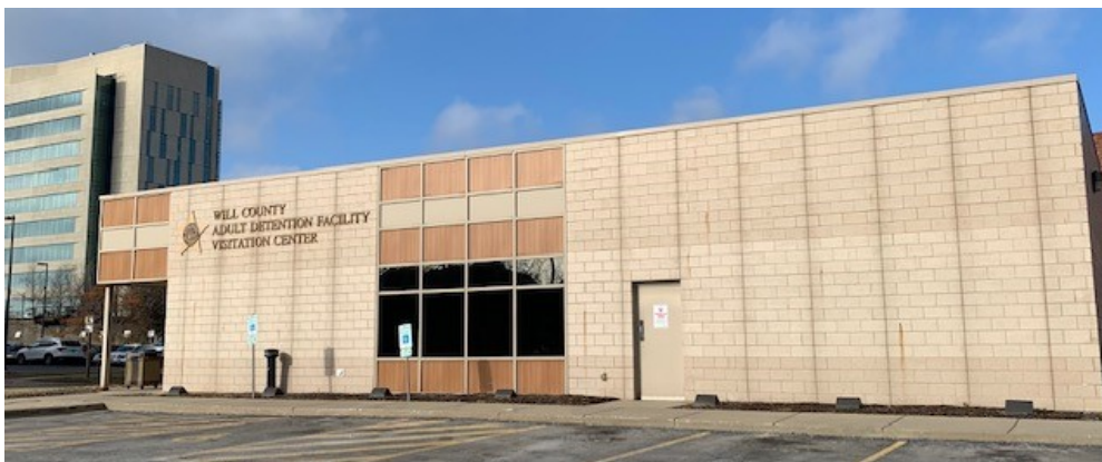
South Elevation at WC Video Visitation Building, 20 S. Chicago St. Joliet, IL
